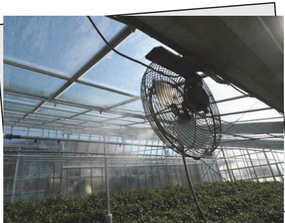
TecnoCooling fog system works on a pressure of 1000 PSI (70 Bar) and it is designed to produce water droplets smaller than 5-10 microns diameter that, for their dwarfish size remains suspended in the air for a long time producing the fog effect.
